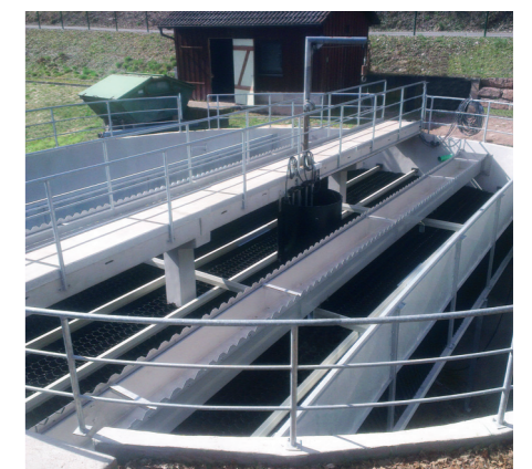
Round tank converted to TUBEdek®
