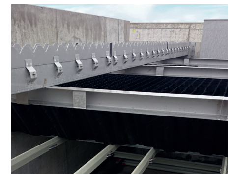
TUBEdek® with support structure and launders
