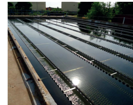
Drinking water plant upgrade
