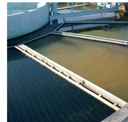
Front left segment with TUBEdek® (remaining segments without)
