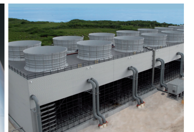
Cooling tower installations
