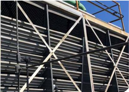
Factory-Assembled, Crossflow Tower Repack
